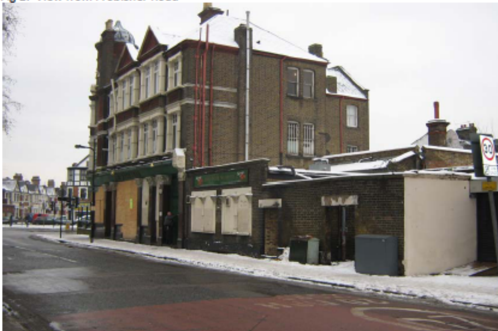
Fig 2: View from Frobisher Road
